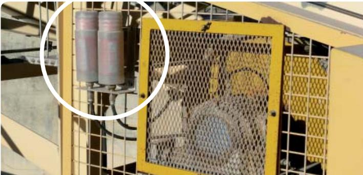
The remote installation of **perma STAR VARIO** lubricators to this conveyor pulley bearing at a cement plant has allowed the hole in the guarding to be repaired. The lubricators can be inspected and serviced safely while equipment is running which has improved safe work practices and saved time.
