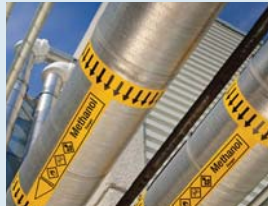
DIY Pipe Marking
